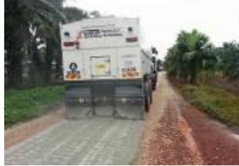
Cement Spreading
