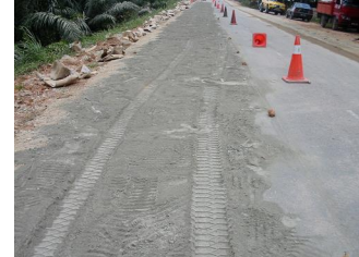
Cement uniformly spread
