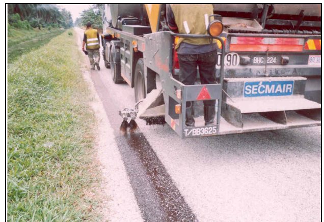
Chipseal work in progress at Parit Bulat, Muar
