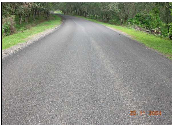
Completed Chipseal work in Felda Jelai FT1279
