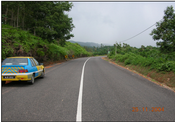
Completed Chipseal work in Felda Bukit Rokan FT 1276
